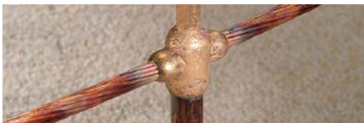
Example of Apliweld Welding for cable to ground rod
